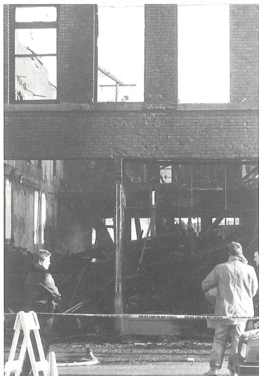
Police and firefighters look over the Bloomfield Building remains.
